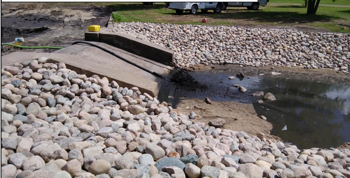
Slurry of muddy water being pumped from the pond in Clearbrook
